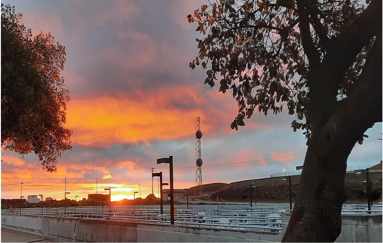
Sunrise at back wash tank at Polonio Pass Water Treatment Plant February 2022
