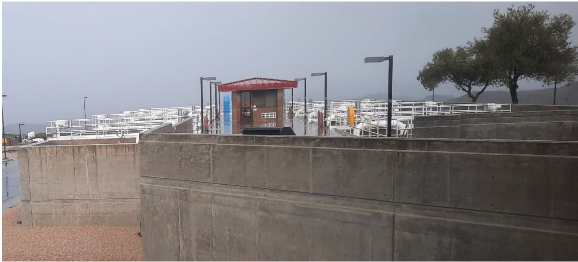
Water Treatment Plant February 2022
