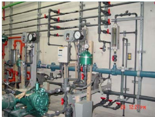
Chemical feed room piping upgrade at the Water Treatment Plant
