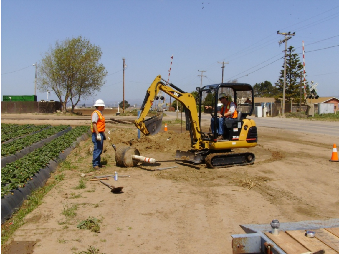
Cathodic Test Station Repair at Black Road
