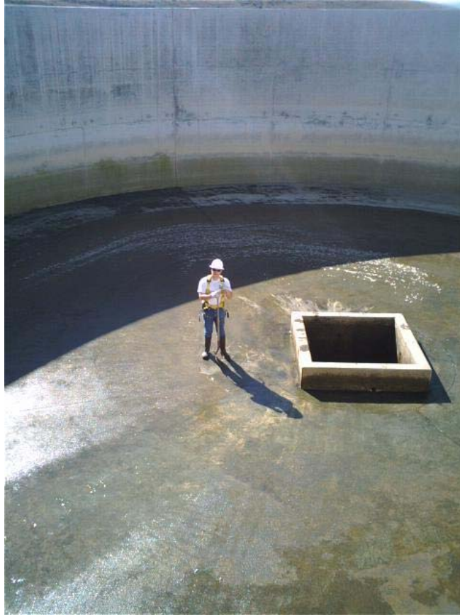
Cleaning of Clear Well at Water Treatment Plant
