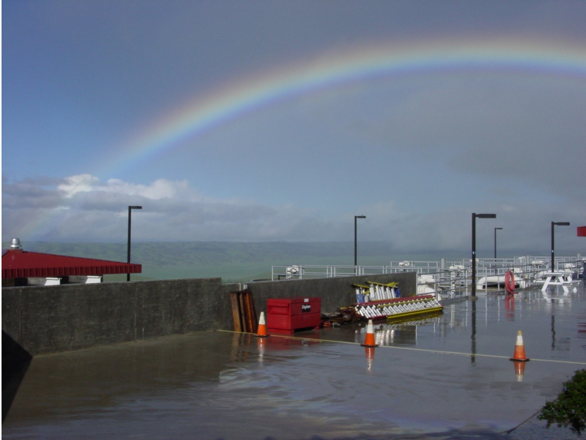
Rainbow over filter deck at the Water Treatment Plant
