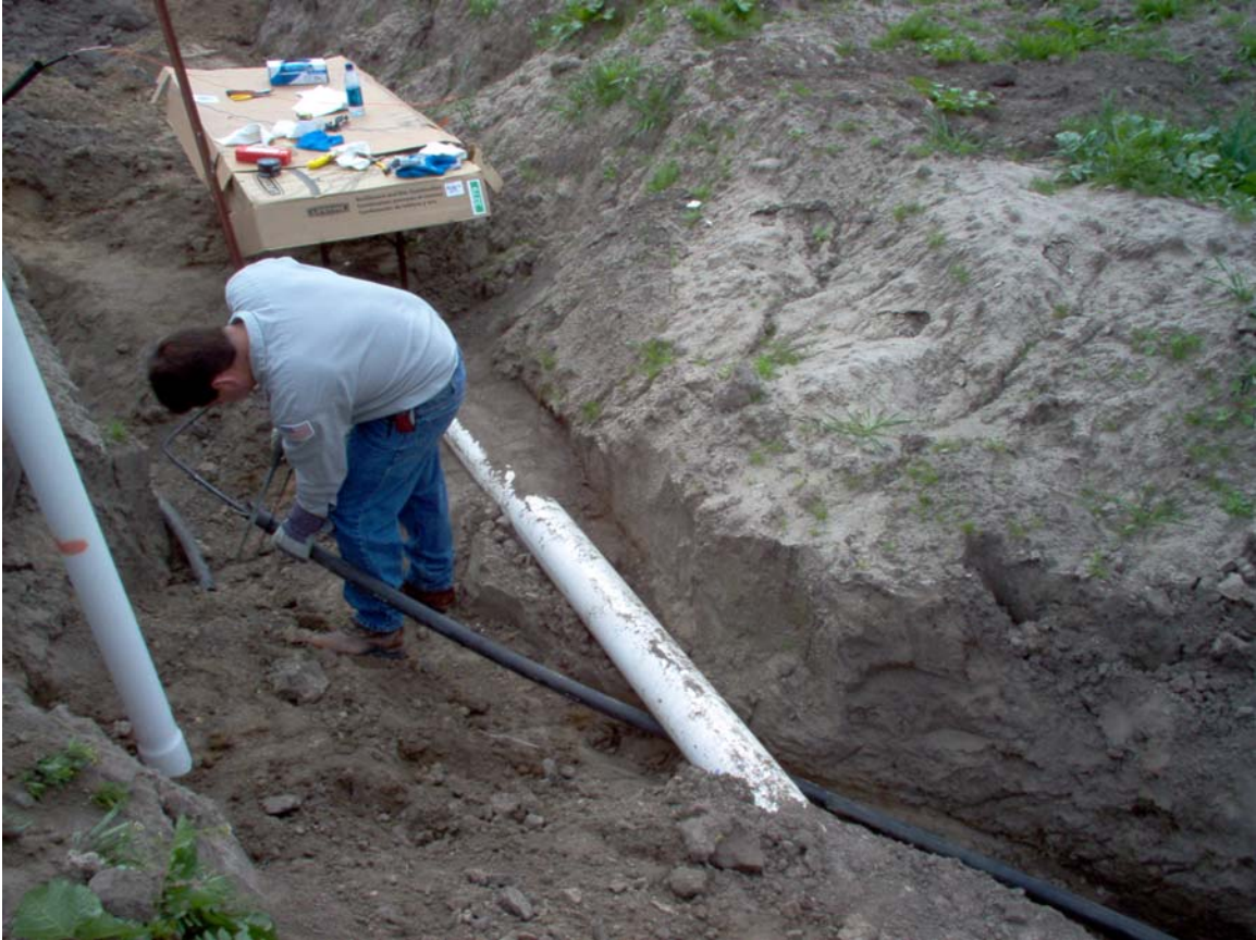
Fiber Optic Cable Repair on Drum Canyon Road
