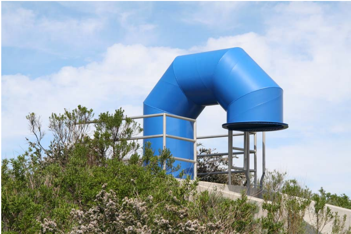
Tank 5 Overflow Structure
