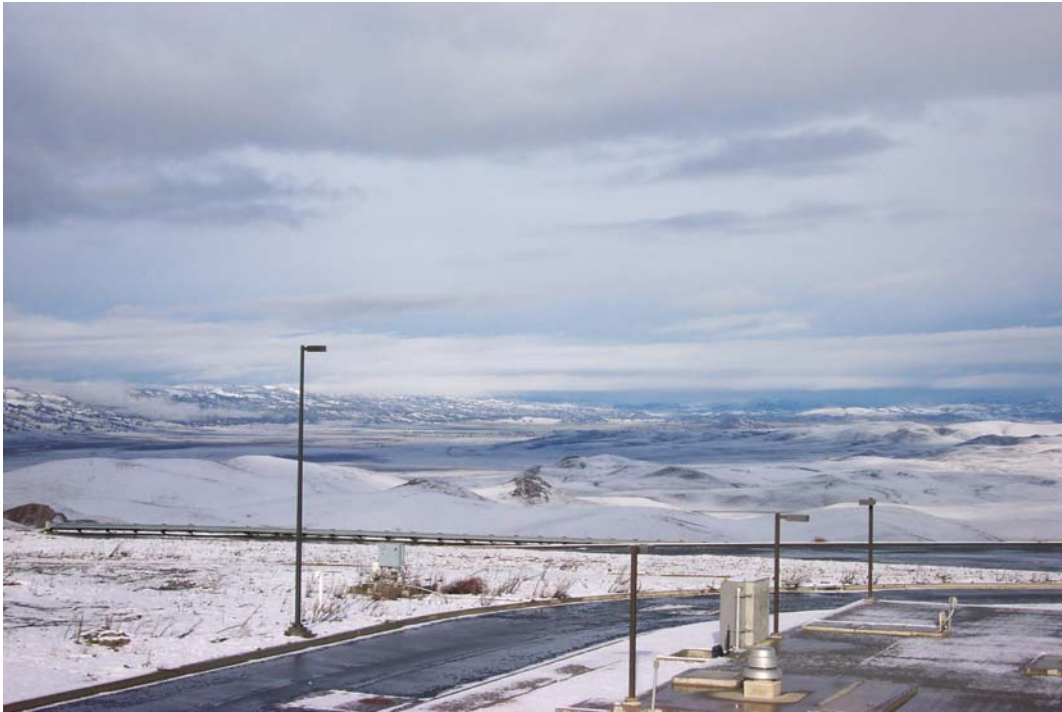
View of Parkfield Valley from Polonio Pass Water Treatment Plant
