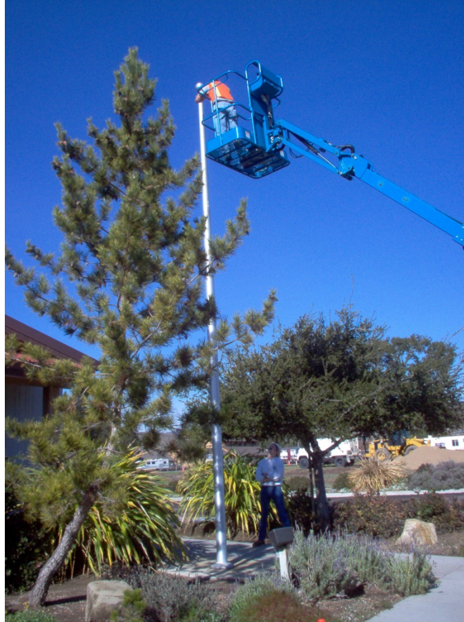
Flag pole repair at Buellton Administrative Office
