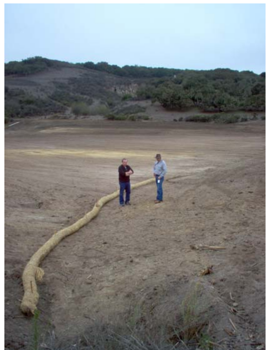
Preparing dewatering area for pipeline leak repair
