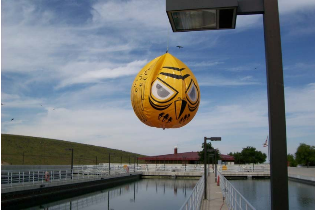
“Scary Eyes” bird deterrent over sedimentary basins at the Polonio Pass Water Treatment Plant
