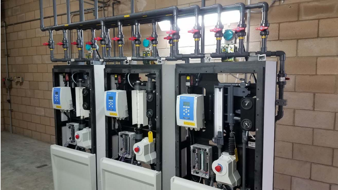
Chlorinators at the Water Treatment Plant installed during Winter Shutdown November 2017
