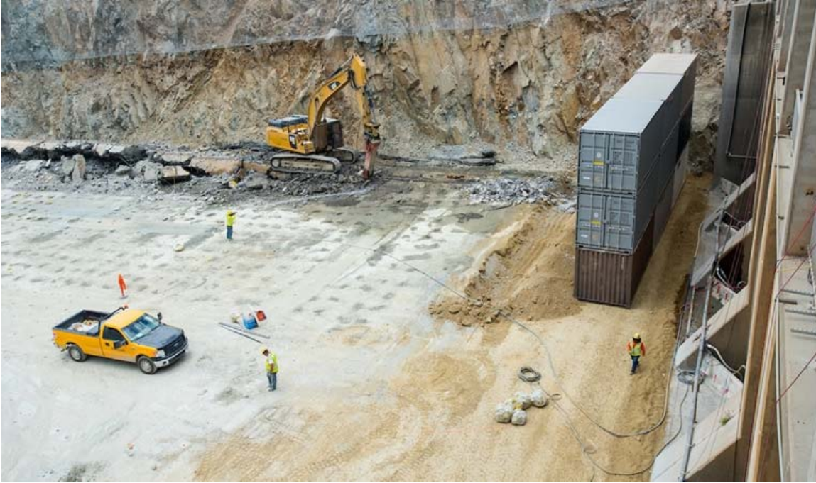
Workers bore a series of holes to contain the explosives for the next round of controlled blasts to break up the original concrete slab of the upper chute of the Lake Oroville main spillway on May 21, 2018. (Photo courtesy DWR)
