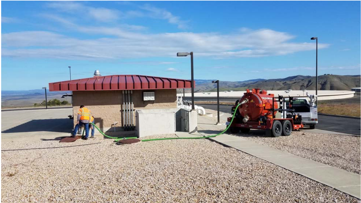
Maintenance clean out of man holes at chlorine contact building at Water Treatment Plant April 2018
