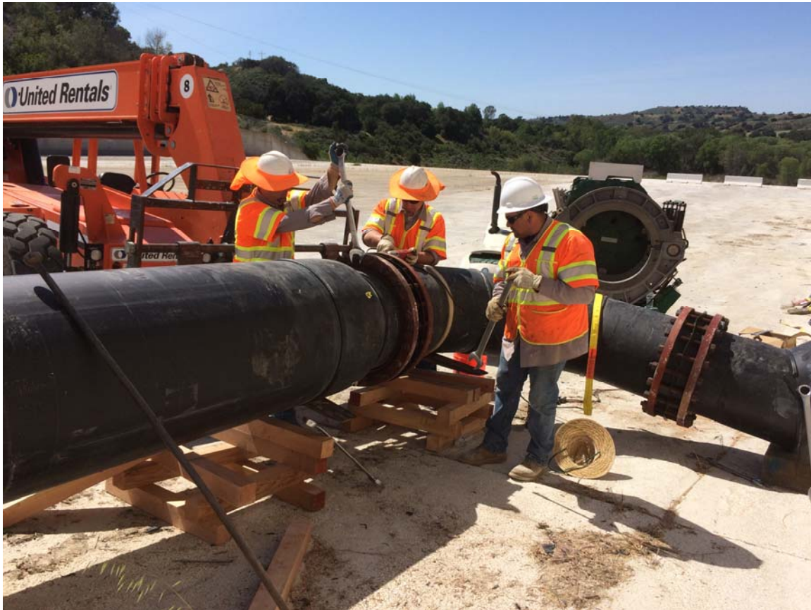
Bypass Pipeline Fusing at Bradbury Dam March 2018
