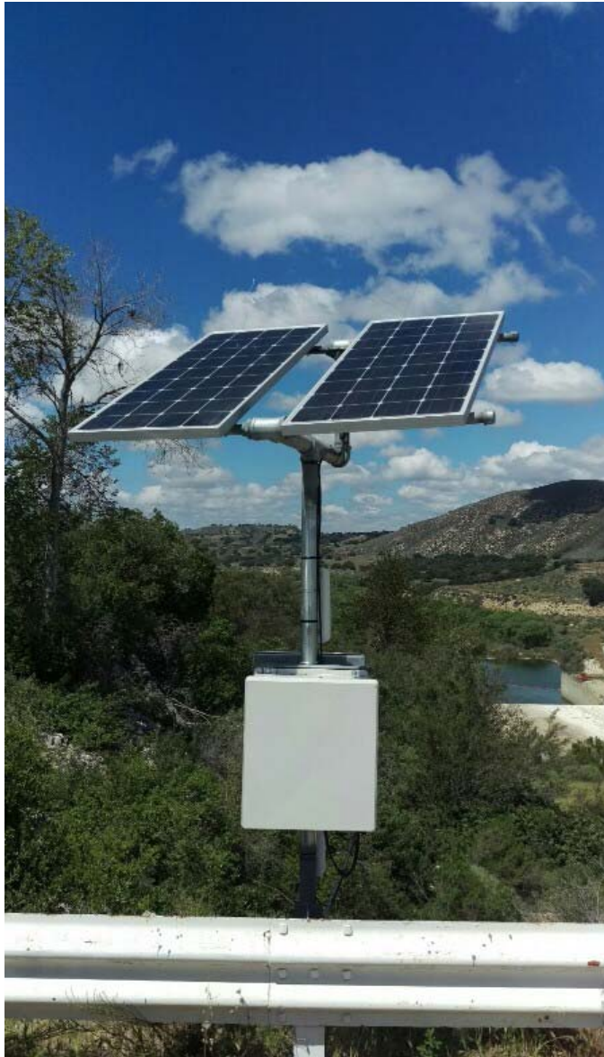
Solar powered repeater unit at Bradbury Dam
