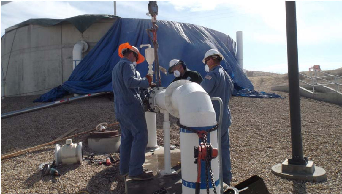
Distribution staff assisting in flow meter replacements at Water Treatment Plant inlet area during Winter Shutdown (November 2017)
