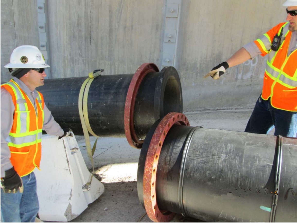
Bypass Piping Reinstallation at Bradbury Dam March 2018
