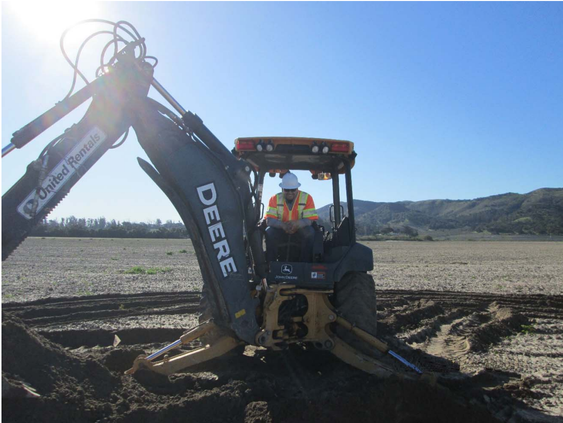
Excavator Preparing for Fiber Optic Repair Work March 2018
