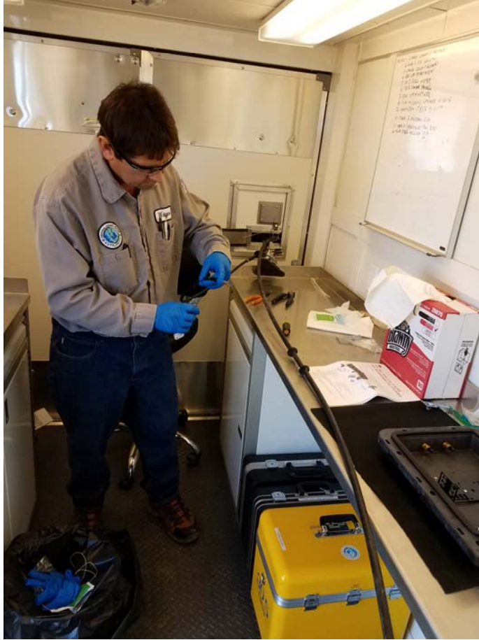
Instrumentation staff performing repair of fiber optic cable break in I&C trailer. April 2018
