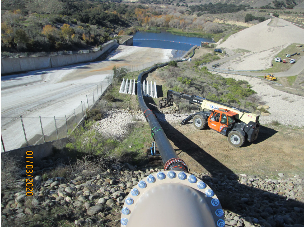
Bypass Pipeline Installation at Bradbury Dam January 2020
