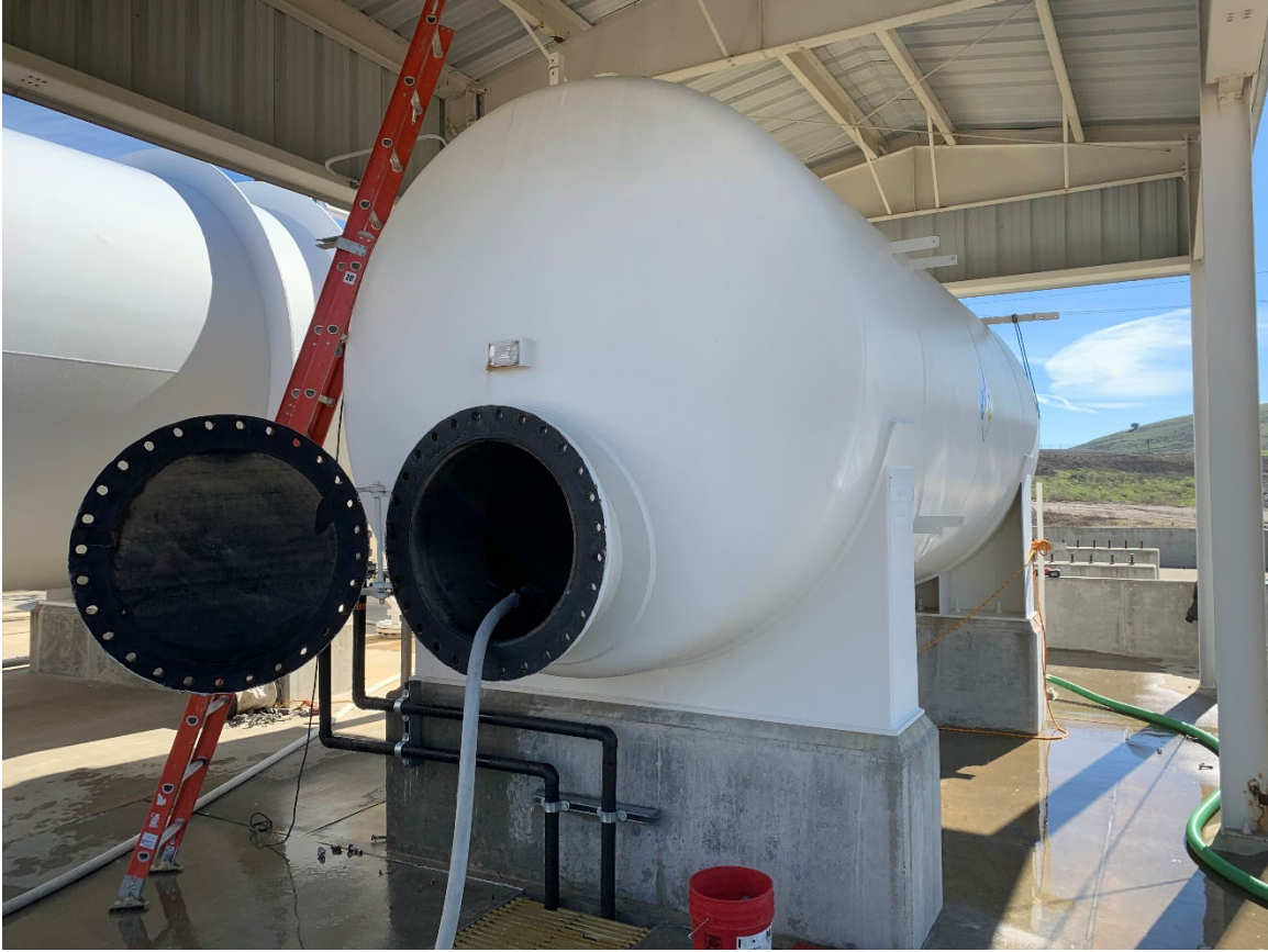
Ammonia tank liner inspection / repairs at the Water Treatment Plant March 2019
