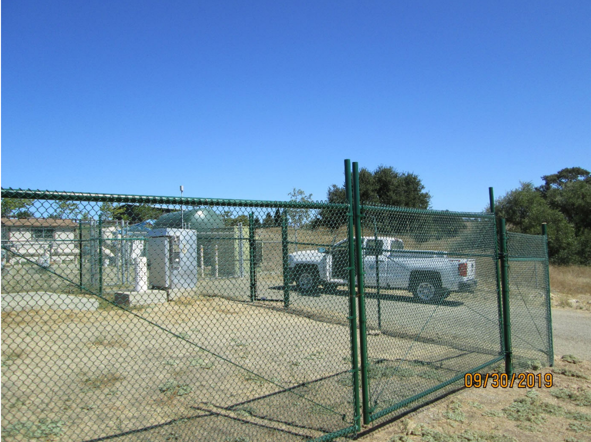
Facility Fencing Project prior to completion September 2019
