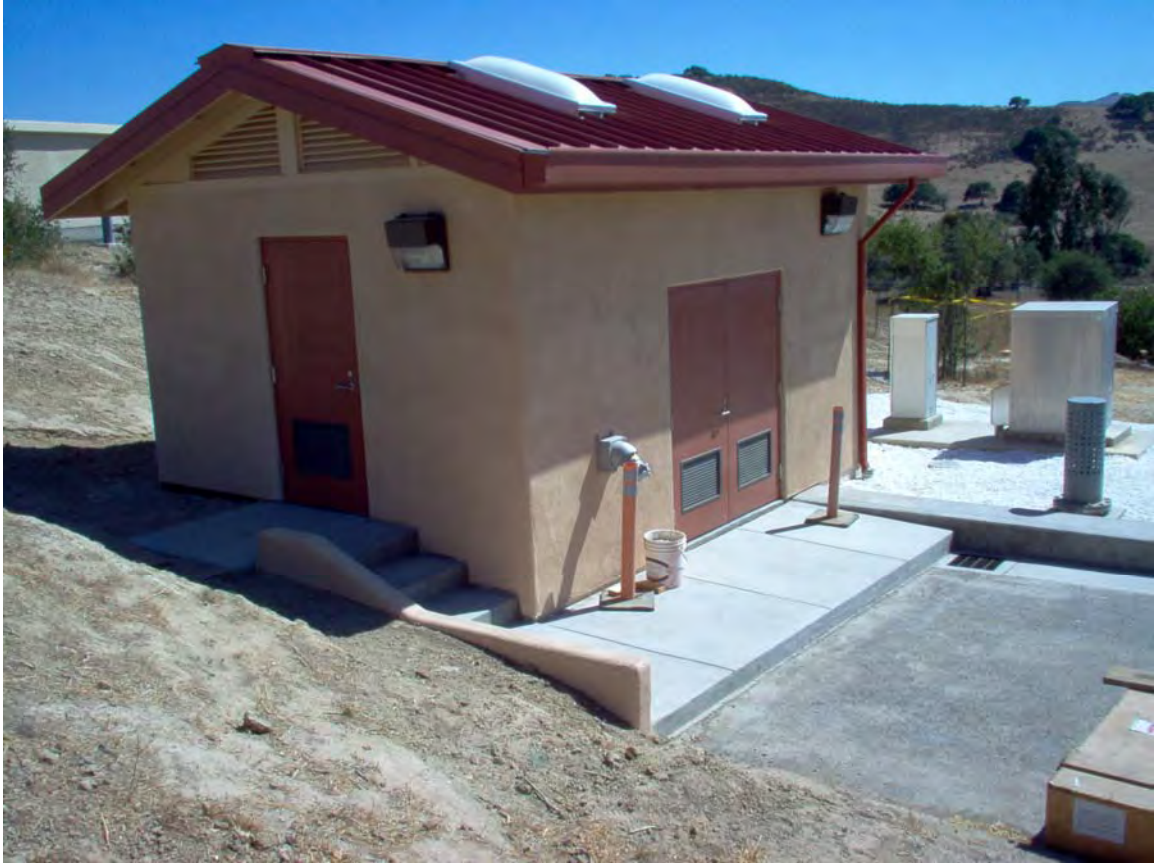
Newly Constructed Tank 7 Utility Building
