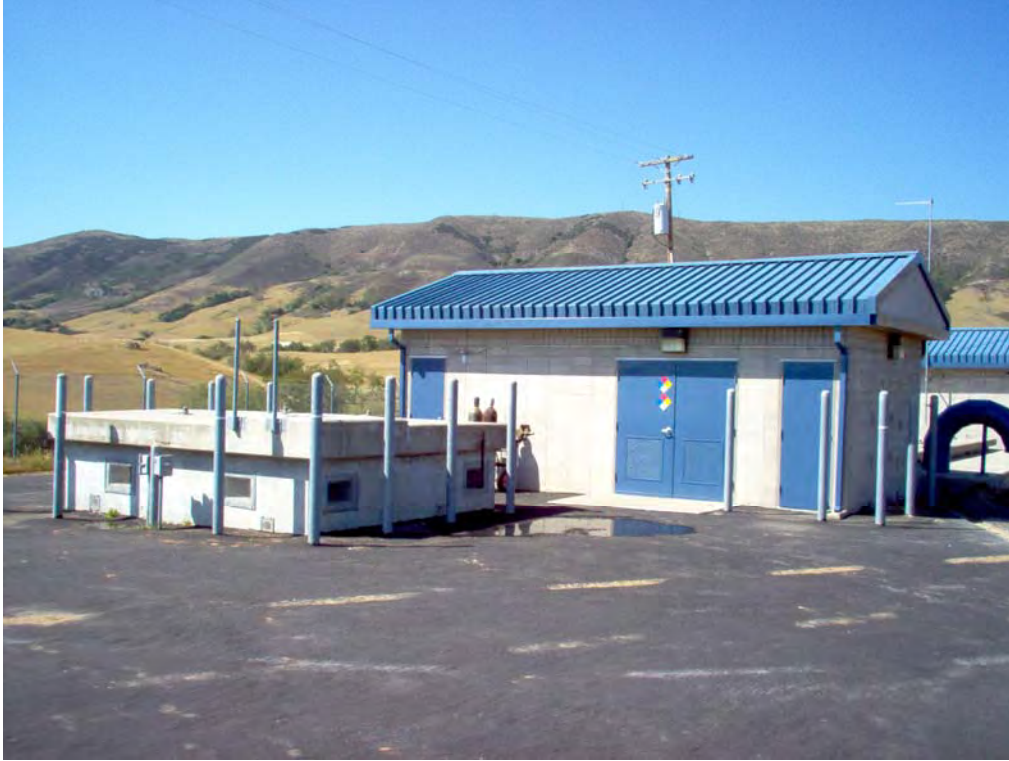
Energy Dissipation Valve Hydraulic Control Building
