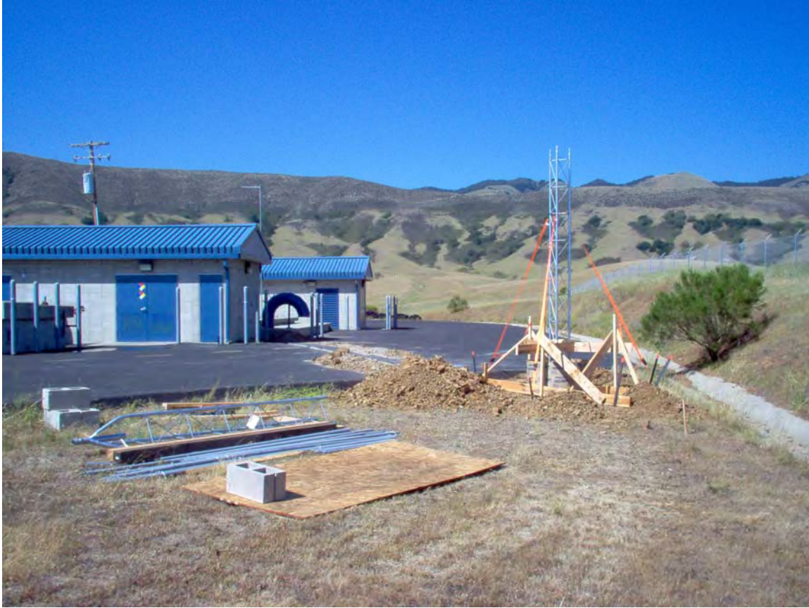
Camera Tower under Construction at Energy Dissipation Vault
