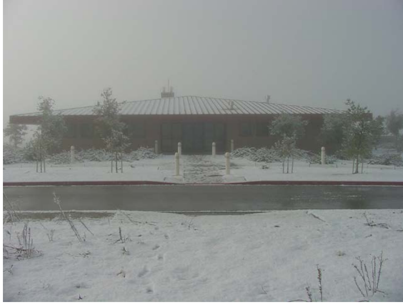
Above: Snowfall at the Polonio Pass Water Treatment Plant.
