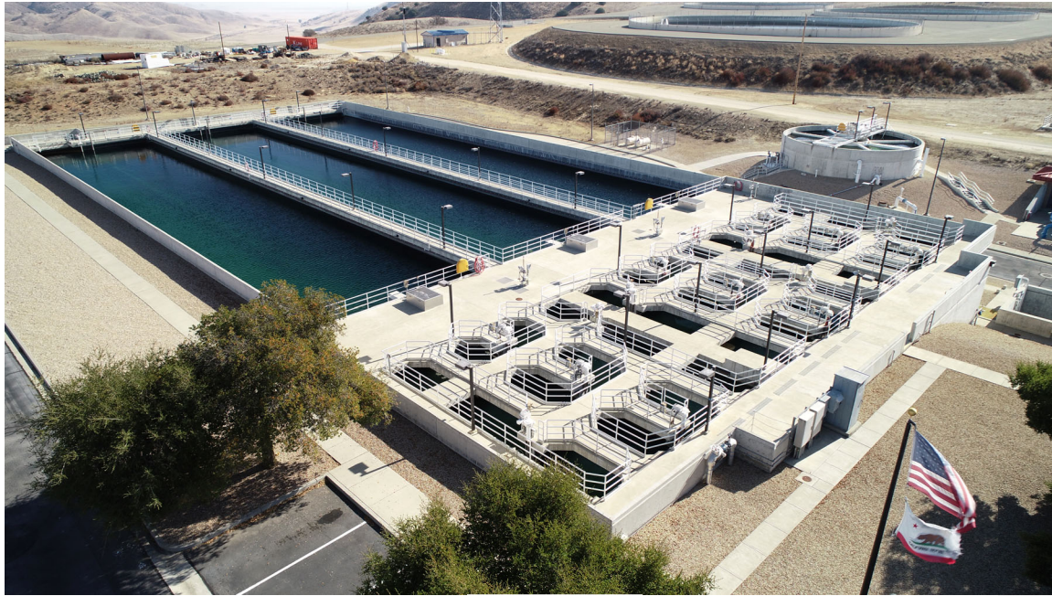
Polonio Pass Water Treatment Plant filter bays January 2021
