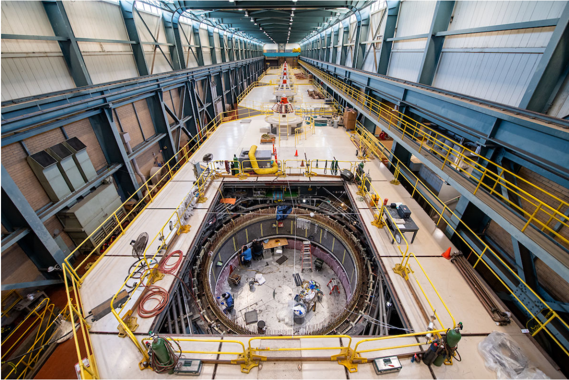
Motor refurbishment work for one of the units in William R. Gianelli Pumping-Generating Plant which pumps water from O'Neill Forebay into the San Luis Reservoir. (Photo courtesy DWR)
