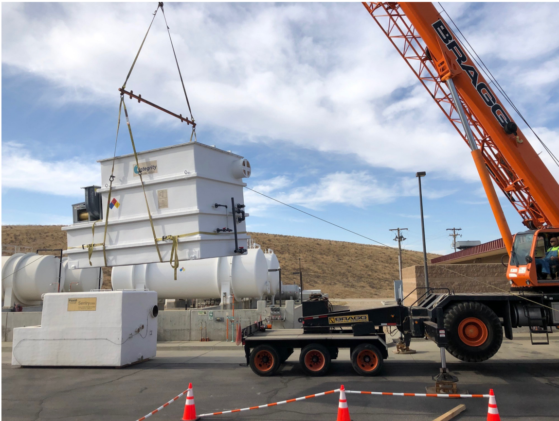
New chlorine scrubber at the Polonio Pass Water Treatment Plant November 2020
