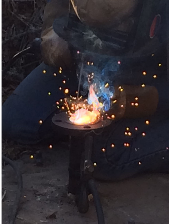
Pipe Riser Repair Project December 2020
