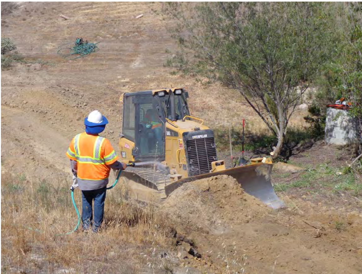
Tank 7 Erosion Repair - June 2014
