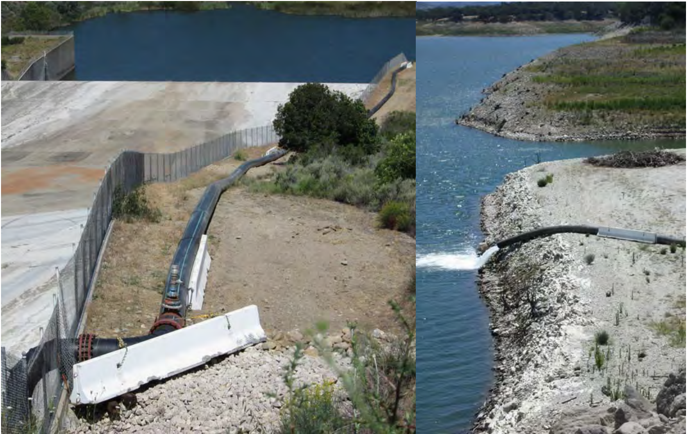
Bradbury Dam Bypass Project – April 2014
