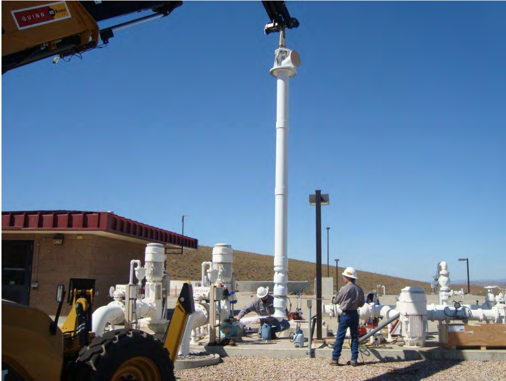
Fire Pump Reinstallation Project
