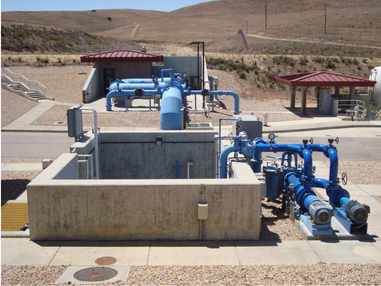
Polonio Pass Water Treatment Plant Flash Mixer with back up pump installed during Winter 2013 Shutdown
