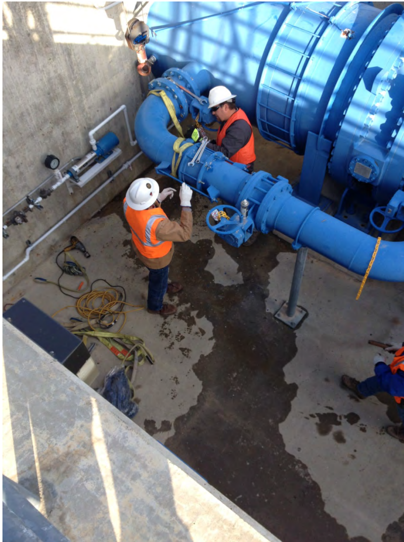
Polonio Pass Water Treatment Plant Exit Vault Investigation – March 2014
