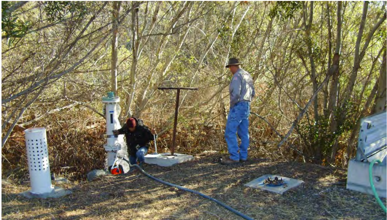
Dechlorinating at Blowoff #1 – Winter 2013 Shutdown
