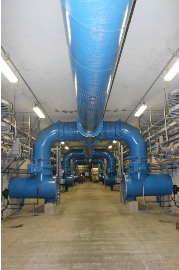
Polonio Pass Water Treatment Plant Filter Backwash Line
