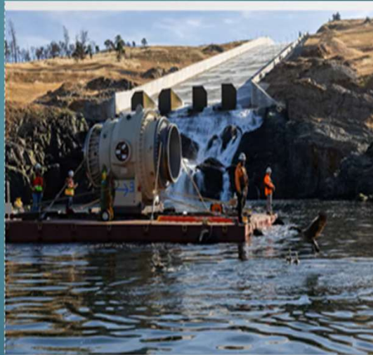
River Valve Outlet System
