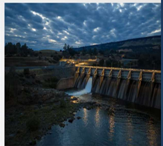
Thermalito Diversion Dam
