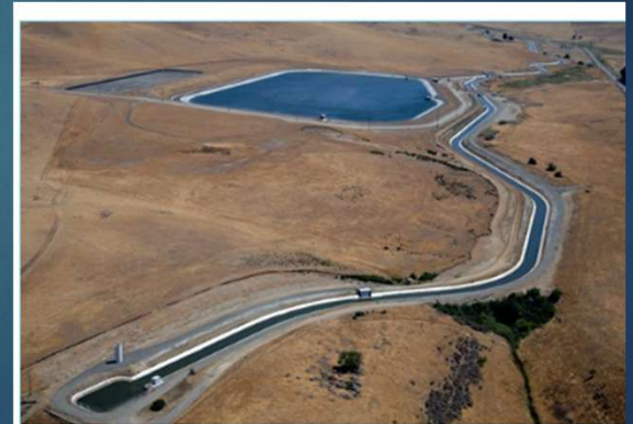
Dyer Reservoir and the South Bay Aqueduct located in Alameda County. DWR/2012.
