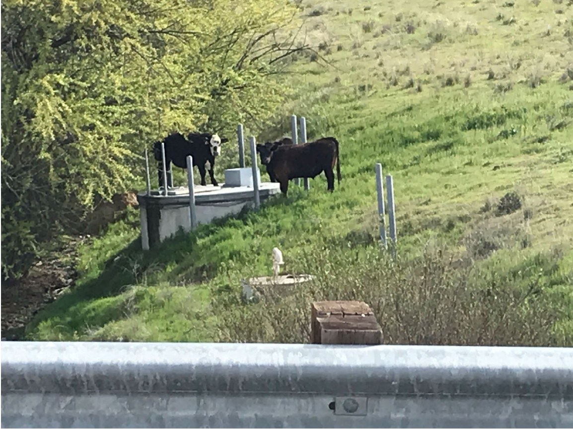
Cattle grazing on CCWA ROW near Polonio Pass Water Treatment Plant
