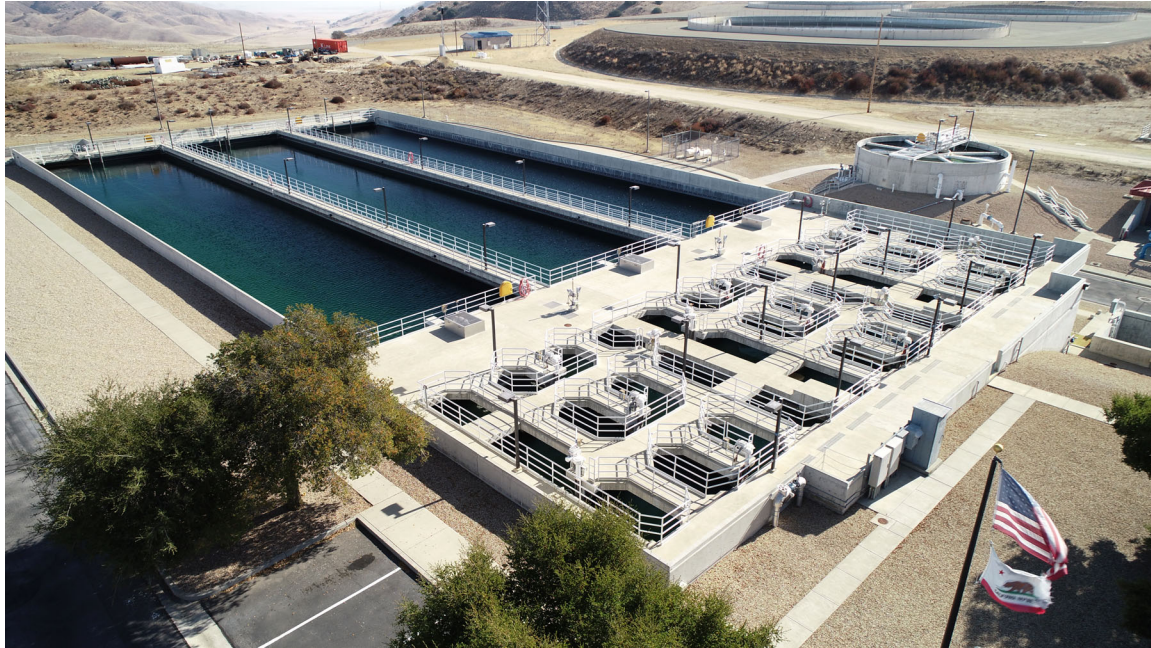
Polonio Pass Water Treatment Plant flocculation/sedimentation basins January 2021
