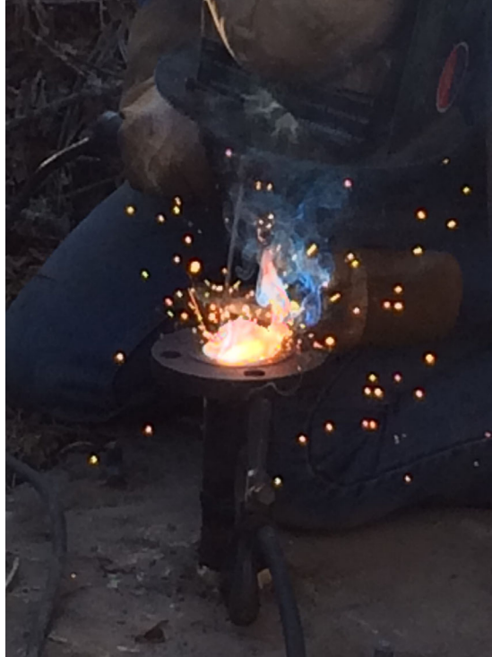
Pipe Riser Repair Project December 2020
