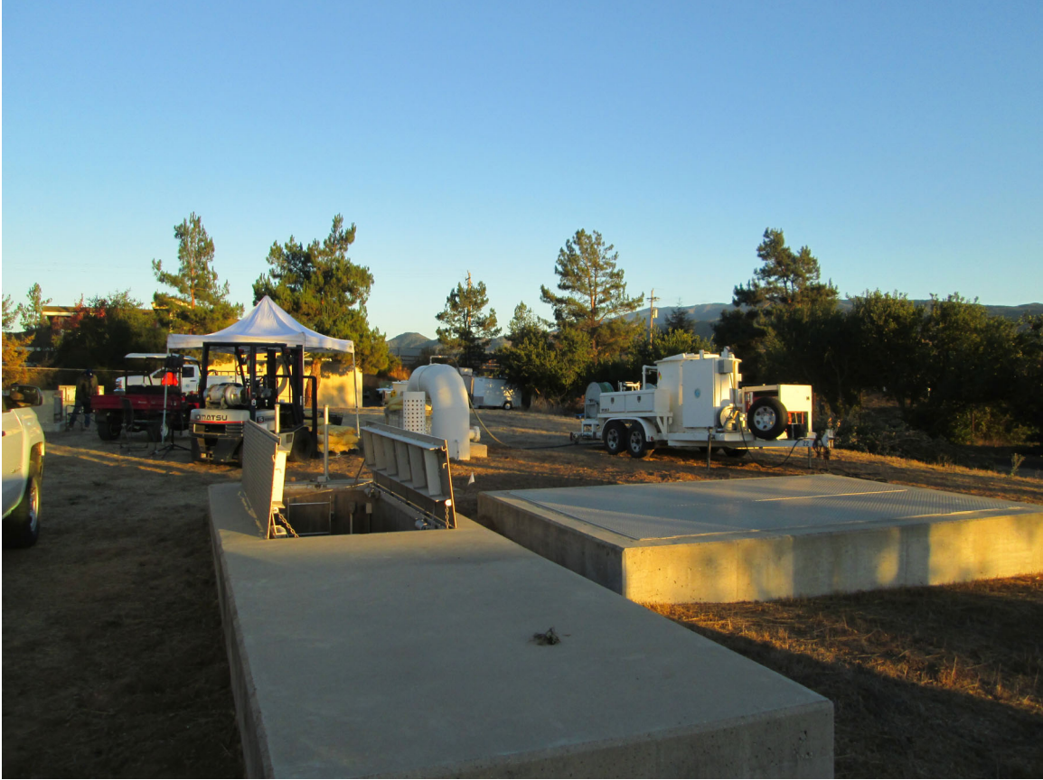
De-Chlorination trailer preparing for injection at Santa Ynez Pump Station inlet vault – November 2020
