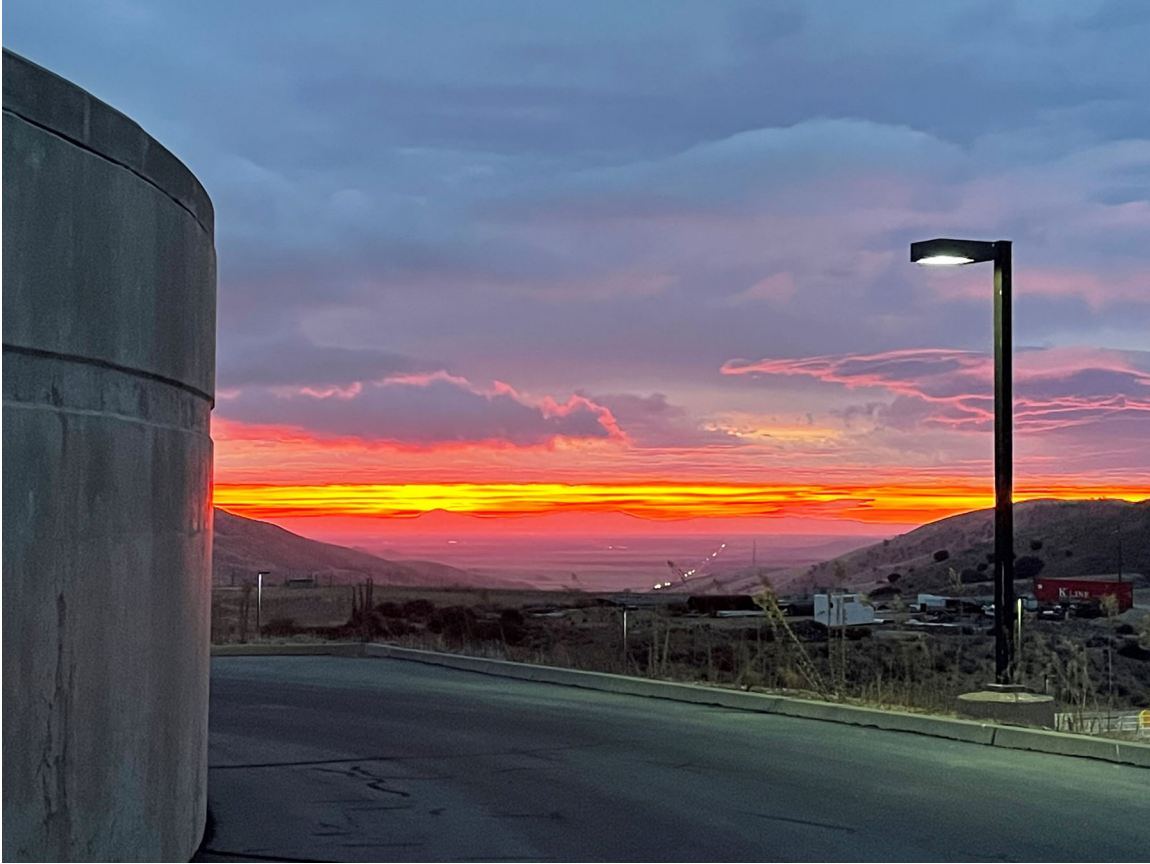
Sunrise at back wash tank at Polonio Pass Water Treatment Plant February 2021
