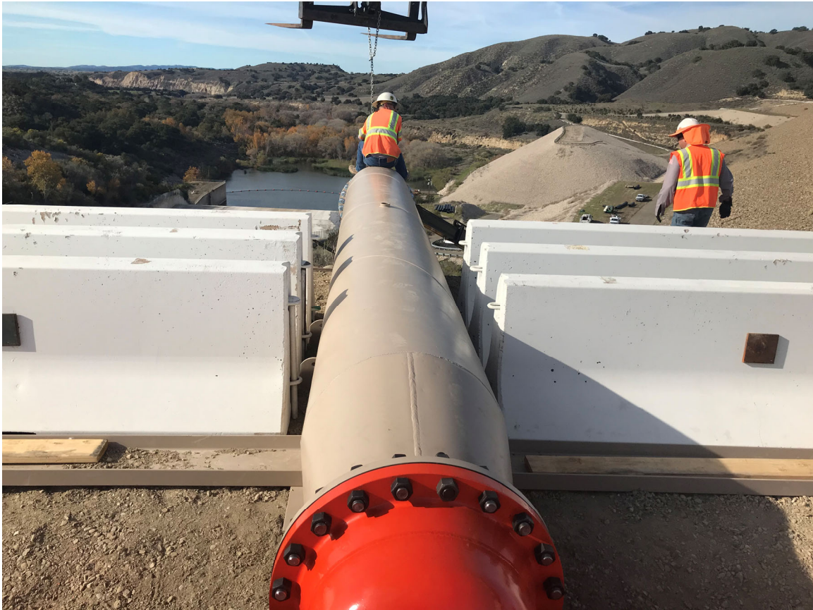
Bypass pipeline connection installation at Bradbury Dam January 2021
