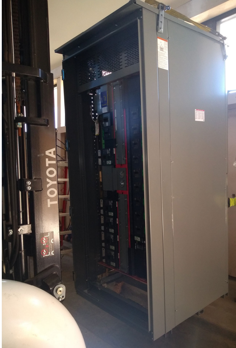
Santa Ynez Pumping Plant Electrical Upgrade February 2021
