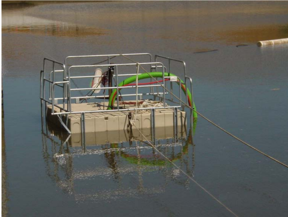
Barge assembly for removal of sediment from Polonio Pass Pumping Plant Forebay.
