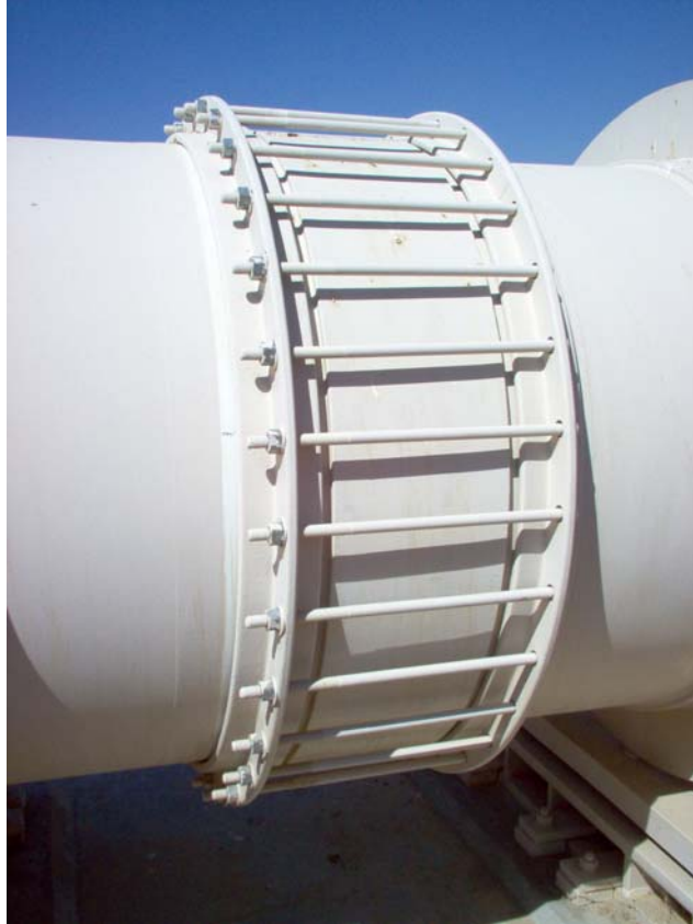
One of 27 flexible couplings at the pipelines San Andreas Fault crossing.
