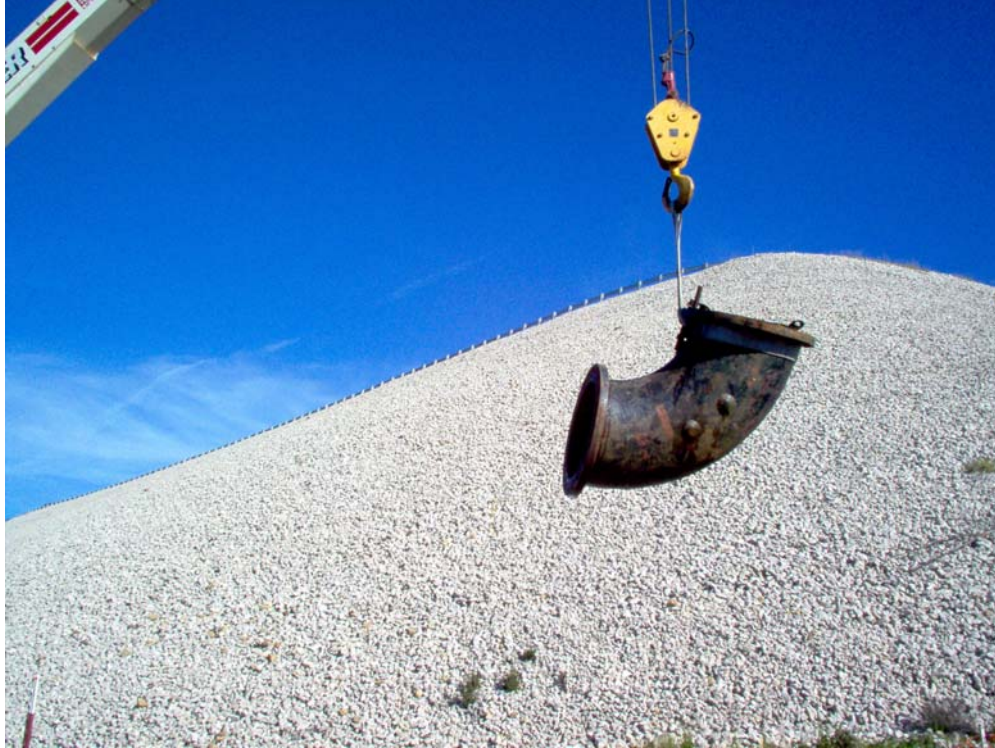
January 2005 removal of temporary pipeline at Bradbury Dam.
