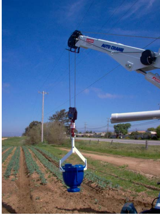
Air Vacuum/Air Release lifting device designed by Tom Petersen, CCWA Distribution Technician.
