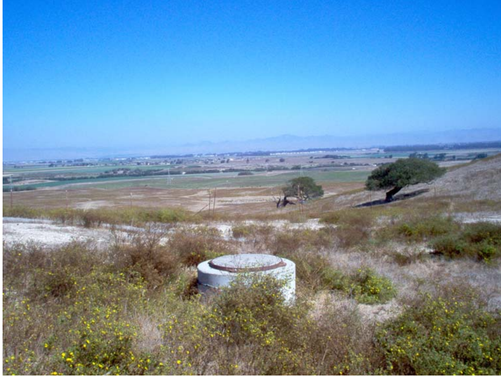
Air vacuum/air release vault overlooking the Santa Maria Valley.
