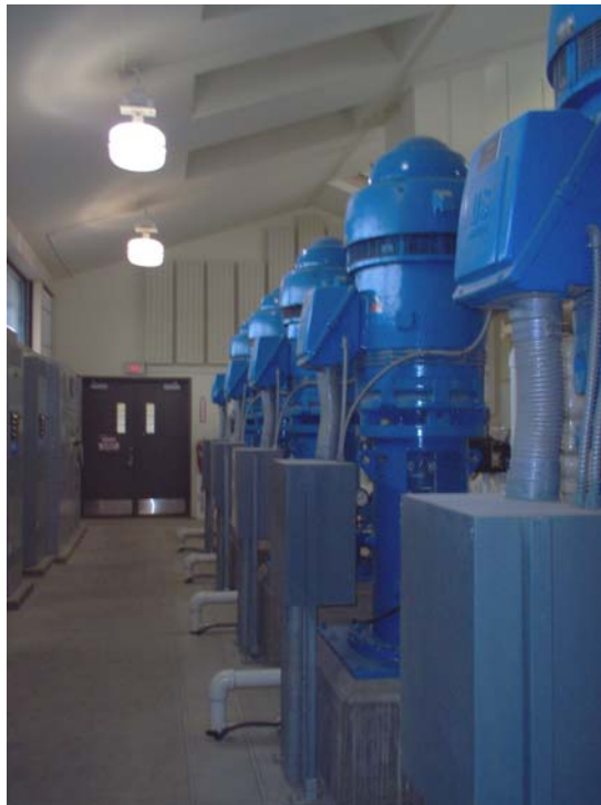
Pump room at the Santa Ynez Pumping Facility.
