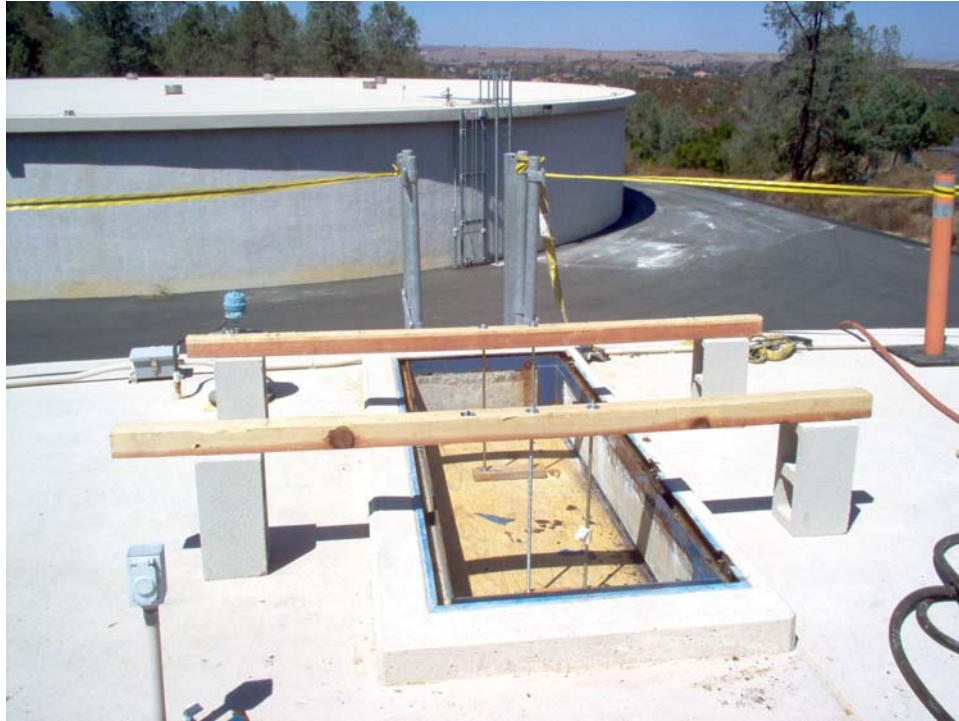
Hatch cover repairs at Tank 2.
