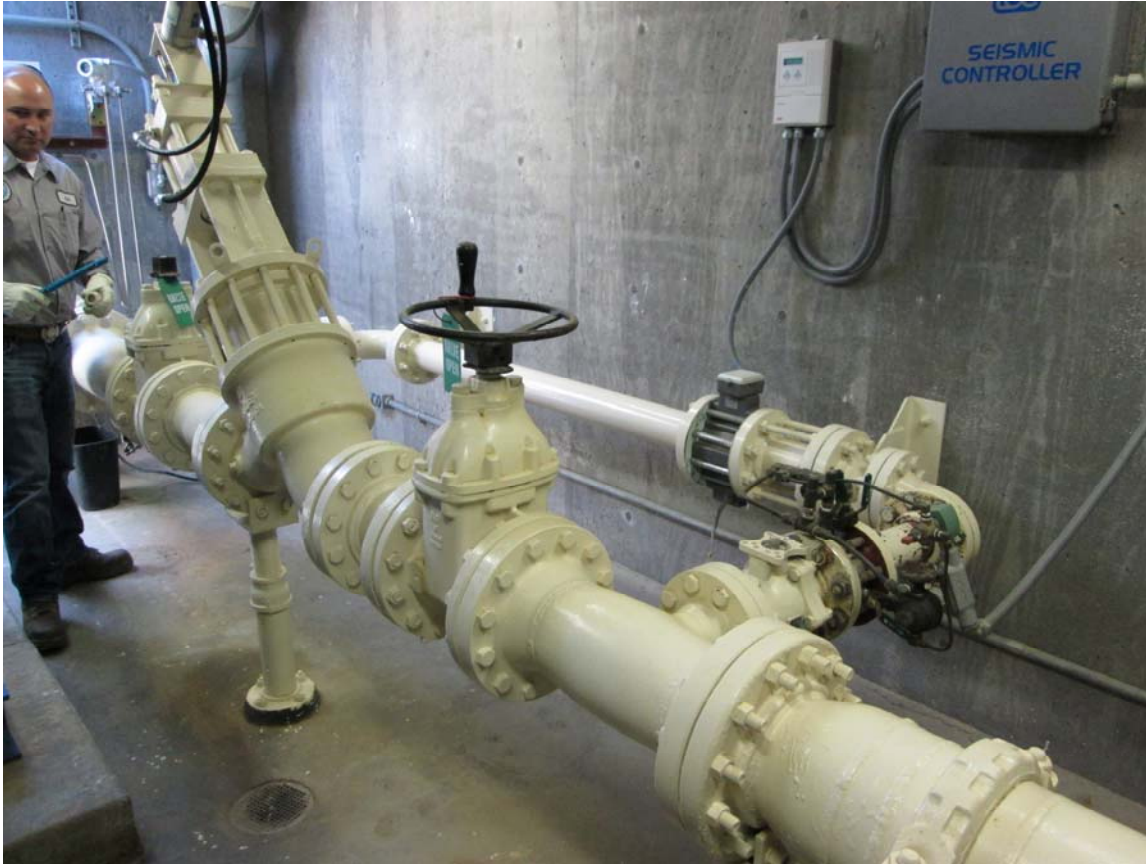
Golden State Water Co. Turnout Valve Operation
