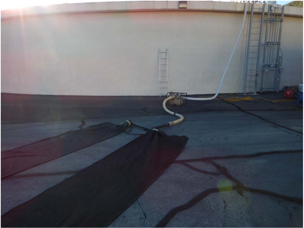
Tank 2 Inspection silt removal system
