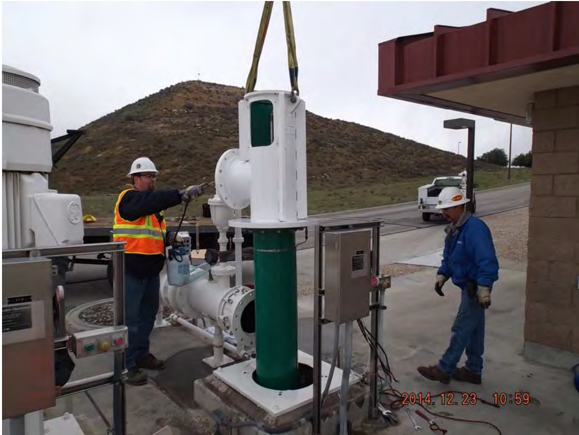
Backwash Pump Installation Project
