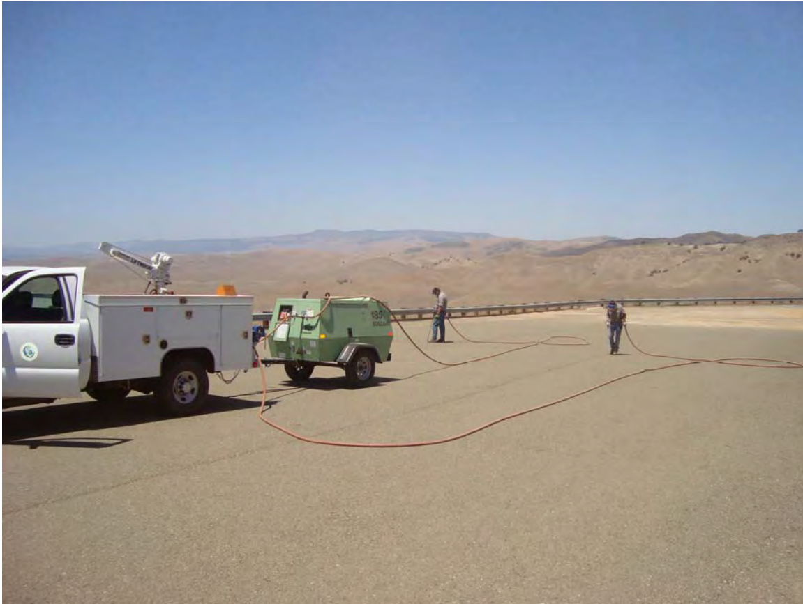
Asphalt crack sealing by CCWA staff at Treatment Plant
