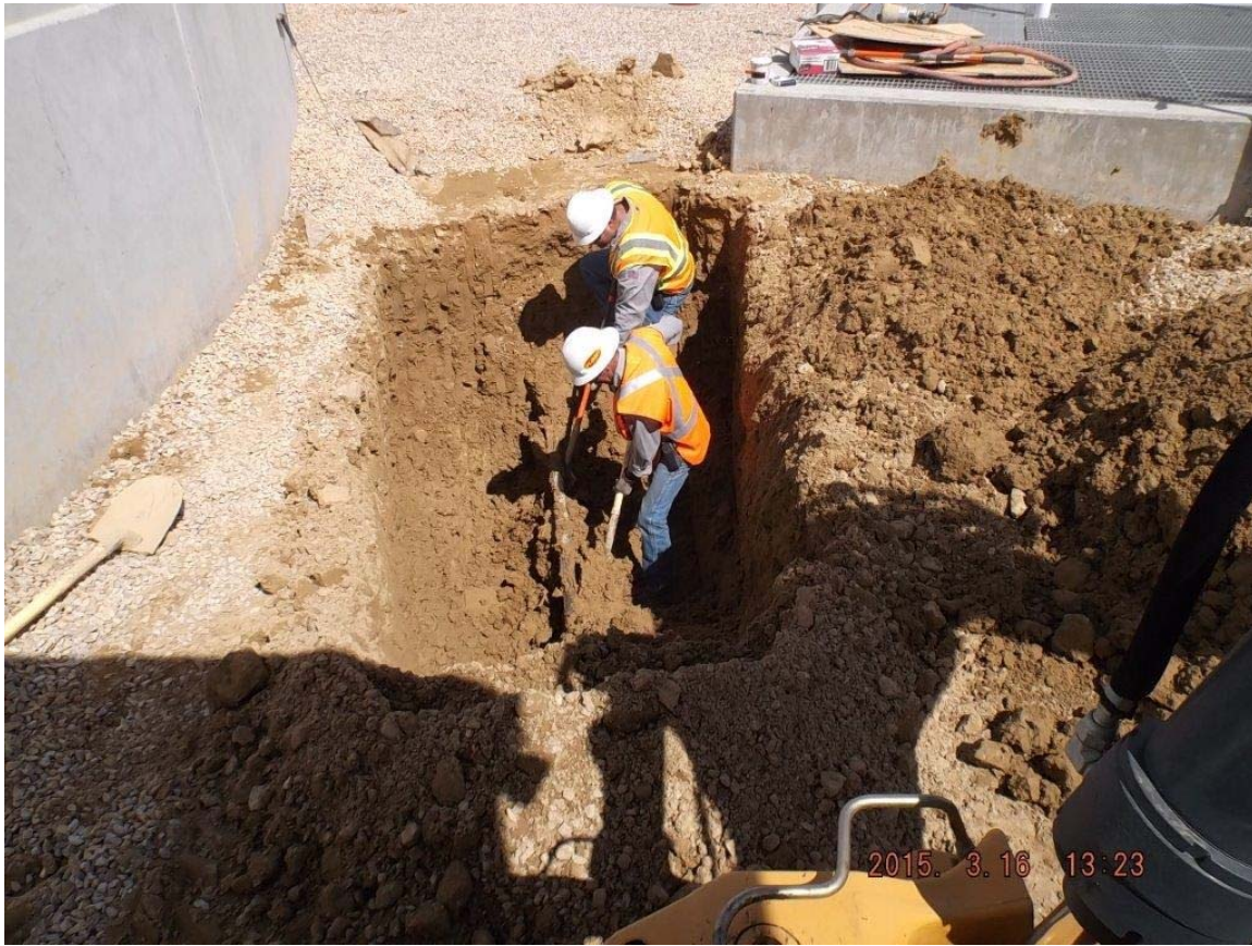
Leak repair at E.Q. Basin at Water Treatment Plant
