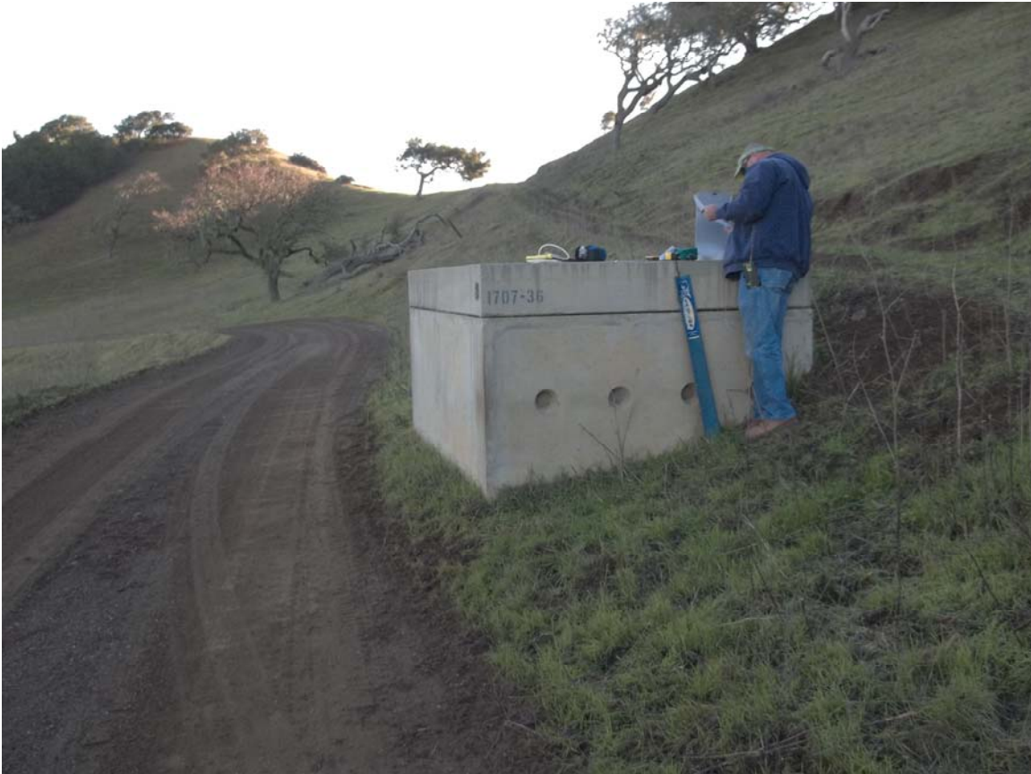
Air & Vacuum vault assessment on SYI line
