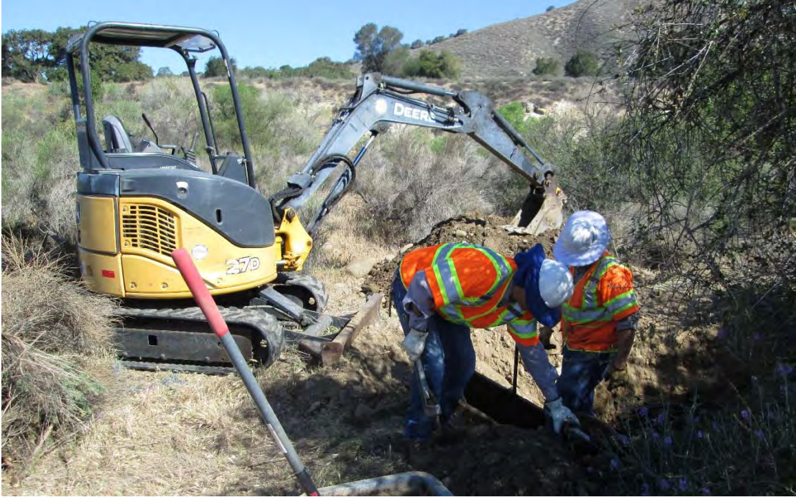
Distribution crew repairing an Air & Vacuum valve on SYII line
