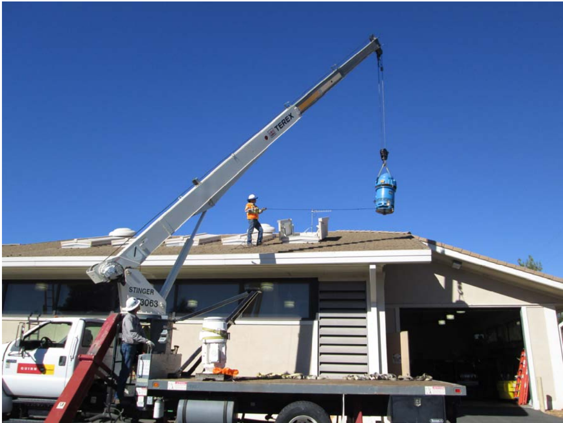
Santa Ynez Pumping Facility Pump Replacement
