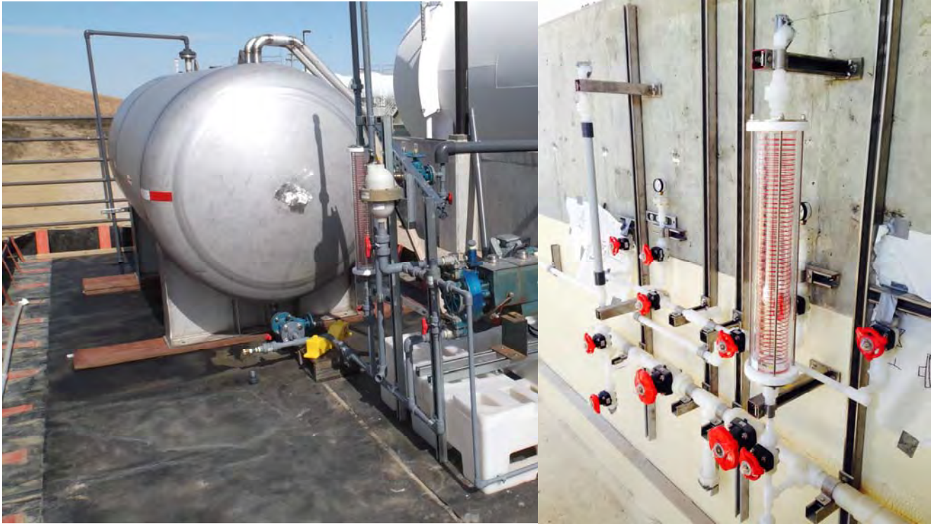
WTP sulfuric acid system piping replacement project
