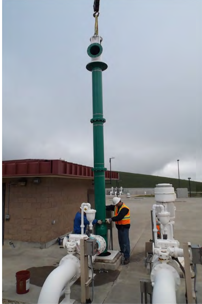
Polonio Pass Water Treatment Plant Backwash Pump Repair
