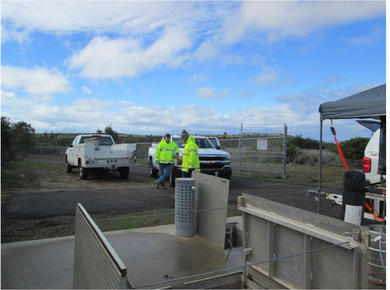
Tank 5 Inlet Vault, February 2022
